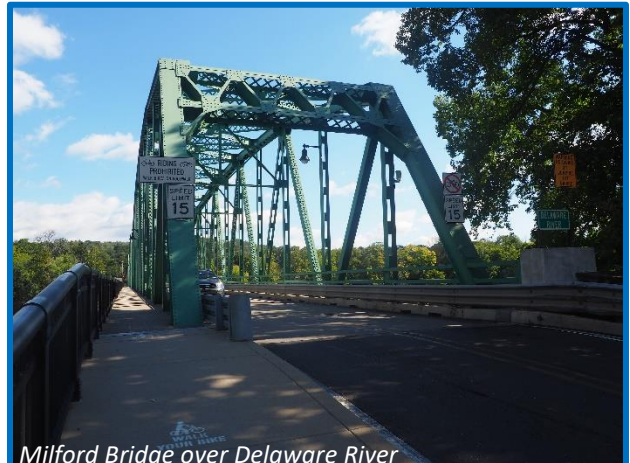
Milford Bridge over Delaware River
